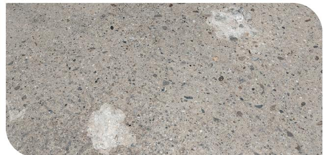
*Example: Properly prepared surface spalls ready for material installation.*
