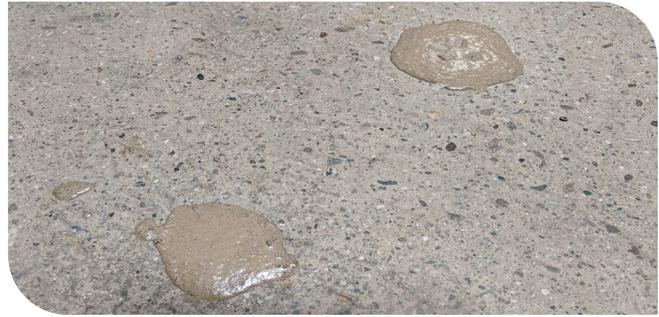
*Example: Slightly overfilled mixed material installed into surface spalls.*
