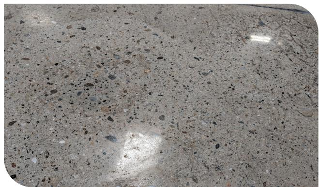
*Example: The filled spalls ground flush to the surface and polished up*
