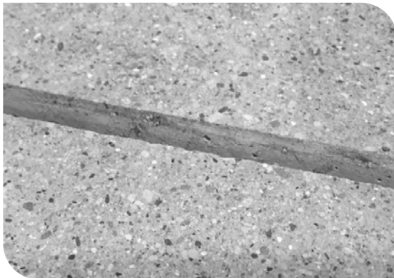
Properly prepared joint sidewalls
