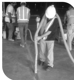
New construction joints being prepared using a vacuum
